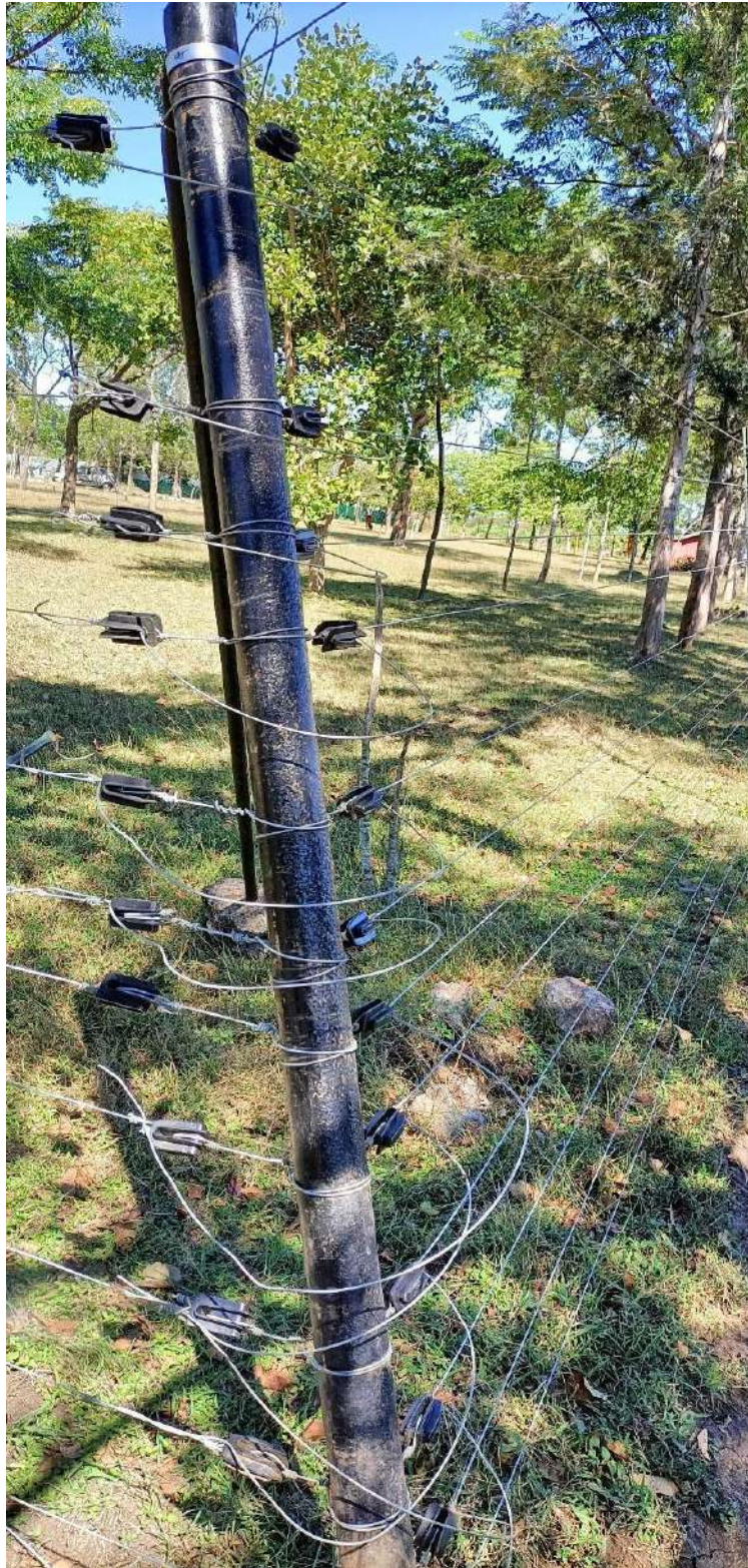
Figure 8 presents a photograph of solar fencing implementation in the Masinagudi range
