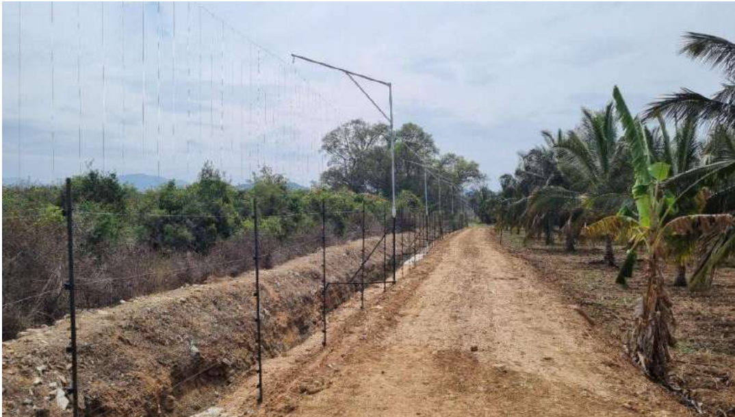
Figure 2. A double-layered fencing system in Thalawady designed for elephant protection
