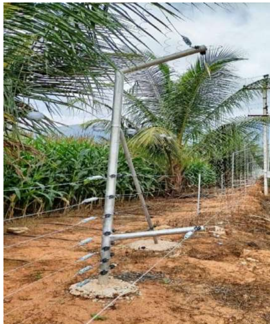
Figure 4. The installatio of Hanging Solar Fencing in the Boluvampaty range
